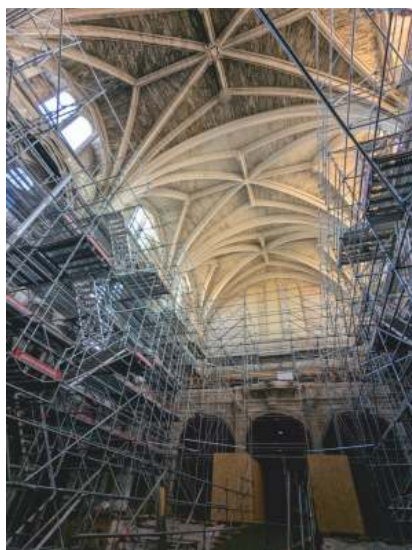
The scaffolding for the first phase of the nave restoration is currently being erected.
